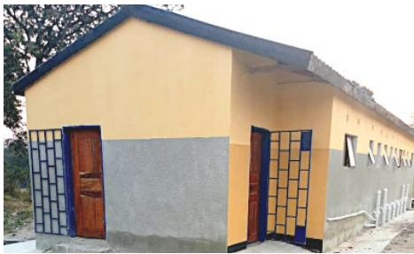
Lavatory exterior complete
