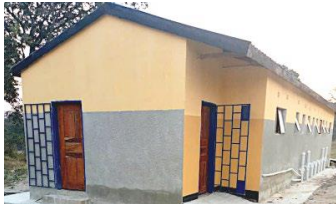
Completed lavatory exterior
