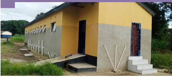
Lavatory Exterior complete
