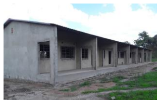
Third classroom complex under roof
