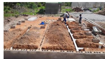
Boys’ lavatory under construction
